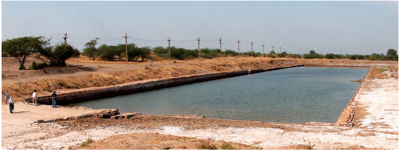
Fig. 6.12. The huge dockyard at Lothal
